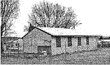
East Street Hall. Rear view. Photo
