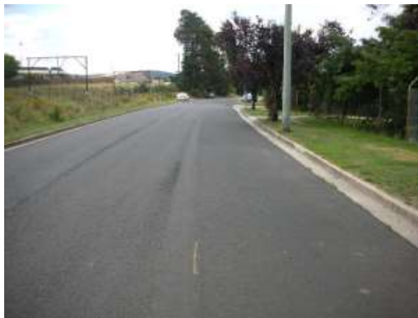
View looking north west along Barton Street subject on right of photo
