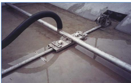
Leopold also offers sludge collection solutions with the Clari-VAC floating sludge collector and the CT2 submerged sludge collector. These systems are used in final clarifiers to remove the sludge solids. For those areas where nitrogen and phosphorus removal is required, Leopold provides elimi-NITE denitrification systems which convert the filters to become biologically active so that the effluent meets the mandated nitrate and phosphorus levels.
