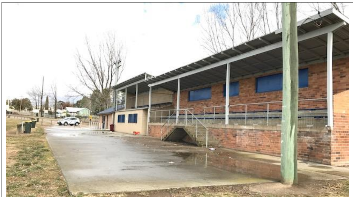
Figure 1 – Lot 2 DP 727021 – Existing Grandstand Facilities to be Demolished
